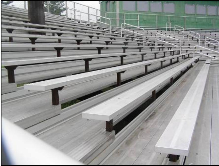
*Newer permanent bleacher system at a town recreational baseball field. The system has aisle railings, riser protection, and top and side guardrails with mesh fencing. The risers should prevent falls between the seatboards and the floorboards and should also prevent objects from falling from the floorboards onto anyone beneath the bleachers.*
