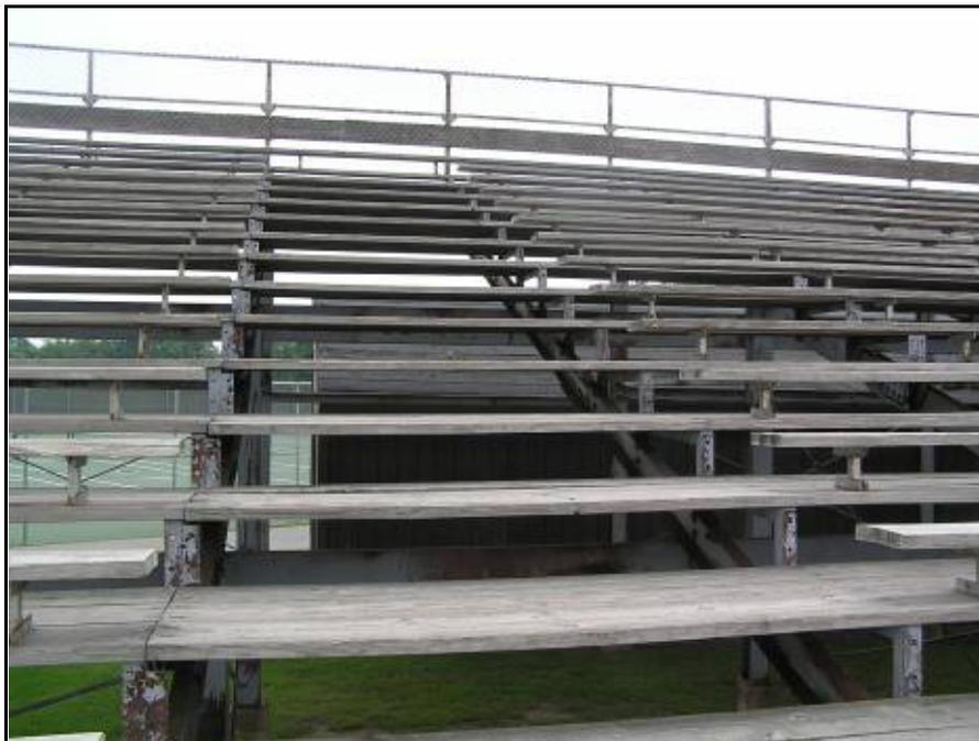
*Older permanent bleacher system at a high school football field. This system has been retrofitted to some degree. There is no riser fall protection and no hand rails in the aisle walkway. However, fencing has been added to the top and sides, reducing the potential for falls from the bleachers. Riser gaps should be closed to reduce the potential for falls between the seat and walking surfaces, especially for children. The installation of aisle railings is recommended.*
